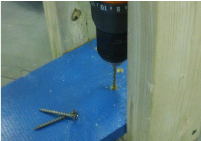
Step 1-8: Drilling the 3/32" pilot holes into the 1x6 (W4), according to the dimensions shown in Figure 2.
