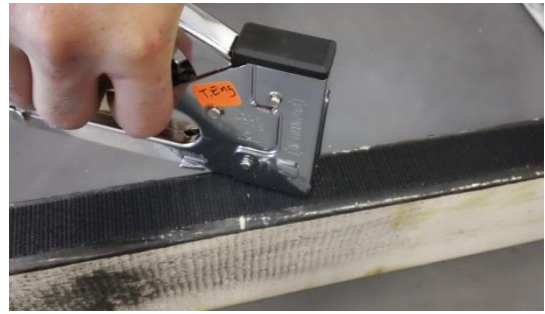
Step 4-1: Use staples to better secure the strips to the crossbeams.
